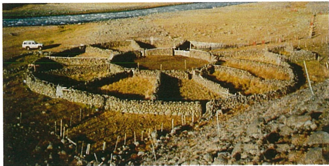
This old sheep corral at Bjarnastaðahlíð in Vesturdalur, called Hlíðar-rétt, is completely made of stones from the river-bank around it. This sheep corral is still in use, every fall. Structures made of stone, without turf can be seen in many places around the country.
