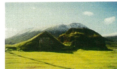
Scattered about Skagafjörður are many turf ruins in which you can see the various techniques used to build and repair them. This picture, taken in 2000, is of the storage shed and smokehouse at Nautabú in Hjaltdalur. When the whole farmhouse was standing, the smokehouse was the open-hearth kitchen.
