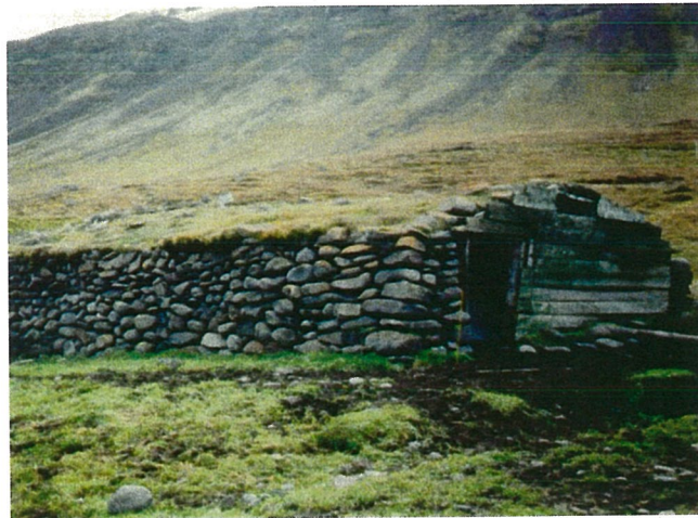
The sheep barns at Skatastaðir in Austurdalur, with two-faced walls built of stone and turf strips. These are primarily stone buildings, but the method of building was to use stone and turf strips alternately, that is, to set each row of stones on top of turf strips all the way up the wall, both inside and outside.
