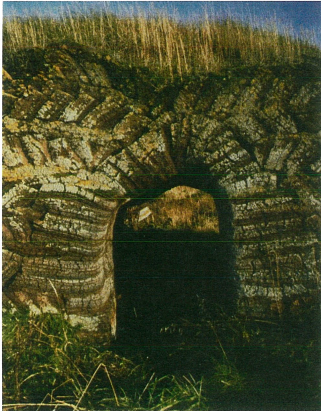
An arched doorway to an animal shed at Krossanes in Vallhólmur. It was laid up out of corner blocks, while the walls are of clamped blocks with strips in between.
