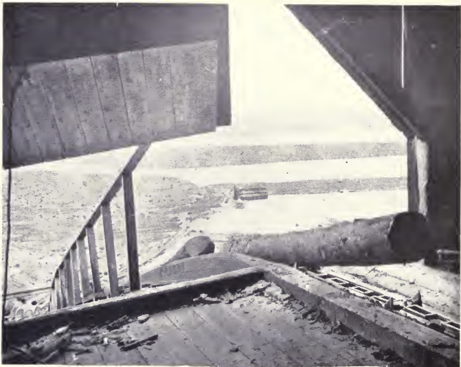
Fig. 36. Jack-Ladder, with Endless Chain.
