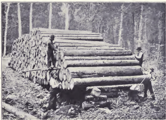
Fig. 9. "Scaling" Logs on the Skids.
