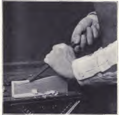
Fig. 69. Paring With a Chisel.
