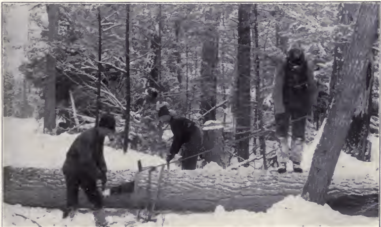
Fig. 6. Sawing Logs into Lengths.
