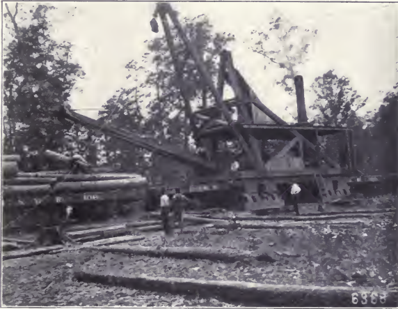
Fig. 27. Steam Skidder at Work. Grant County, Arkansas.
