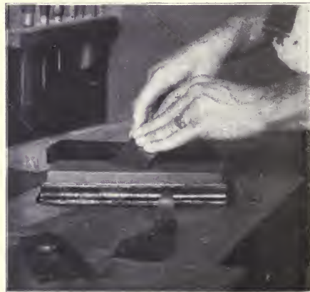
Fig. 77. Whetting a Plane-Bit.
