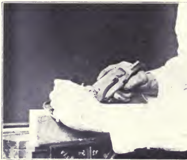
Fig. 272. Thru Chamfering.
