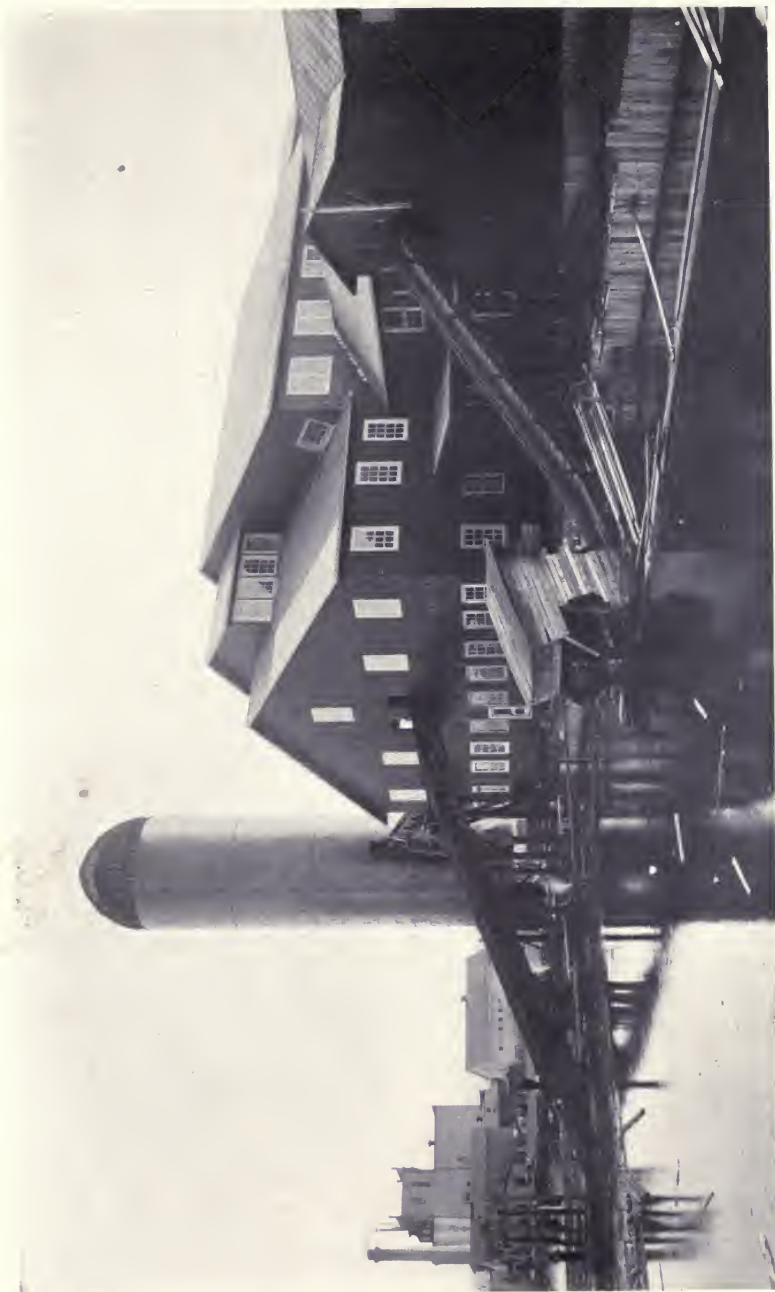
Fig. 37. Two-Story Mill at Virginia, Minnesota, Showing Jack-Ladders and Consumer.
