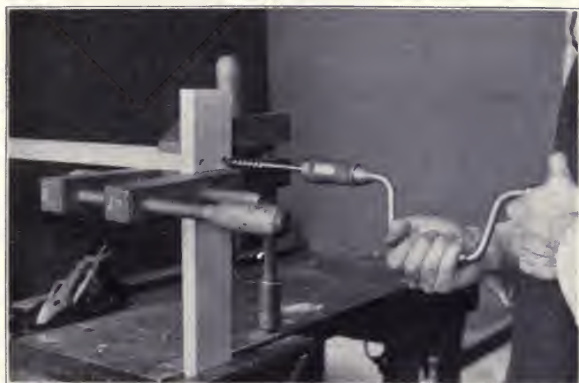
Fig. 247. Thru Boring for a Butt Joint.
