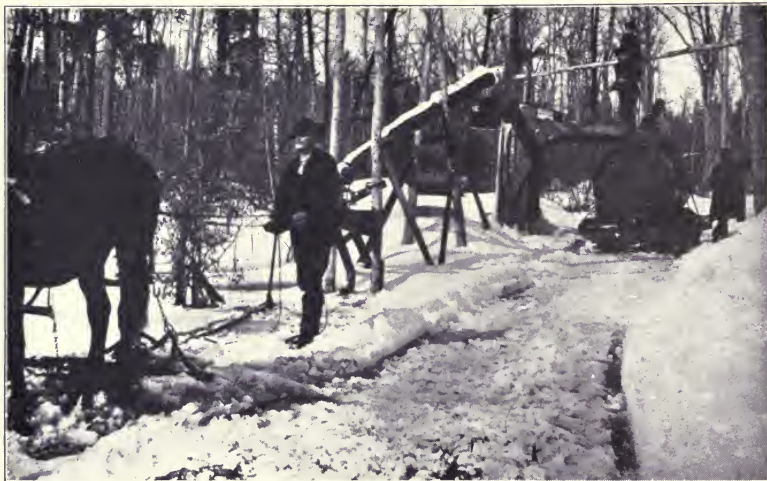
Fig. 10. Making an Ice Road by Flooding.
