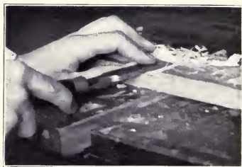
Fig. 71. Chiseling Out a Dado (Second Step).
