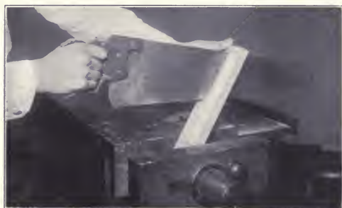
Fig. 89. Rip-sawing with Wood Held in Bench-Vise.
