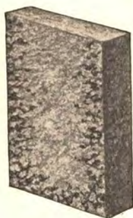
No. 2 Honey-combing Defect.
