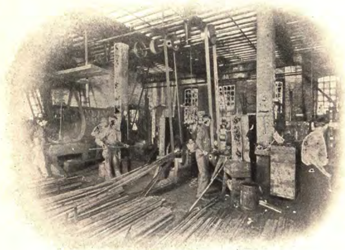
Steel Room, Cutting to Multiples.
