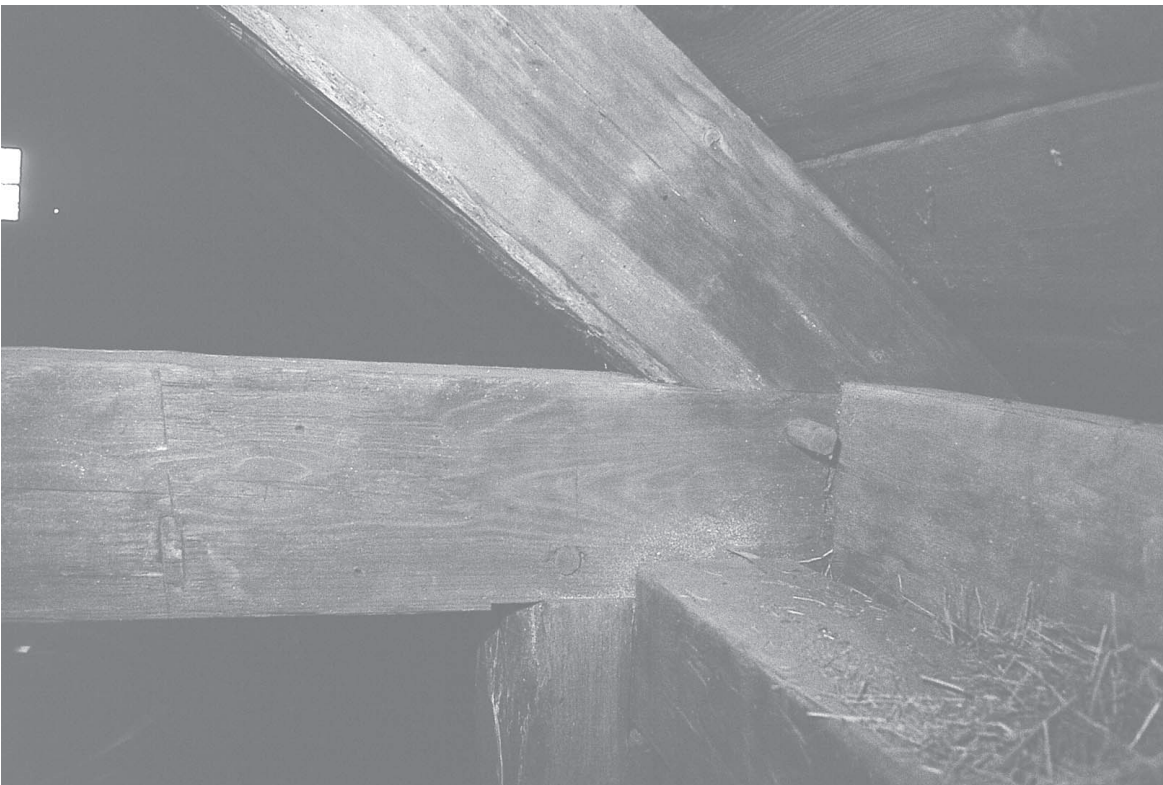
Above, flush tying joints, with top of tie beam and top of plate coplanar, yield neat box frames, as seen in this partly dismantled 1791 house in Cheshire, Massachusetts (see Figs. 11 and 12 of this chapter). Below, mid-18th-century aisled barn in Kensington, New Hampshire, with English tying joint and rare extended tie beams that cross the main, continuous plate and carry the members of an interrupted flying plate tenoned between them. The flying plate, seen to the right of the peg, supports a Greek Revival cornice.
