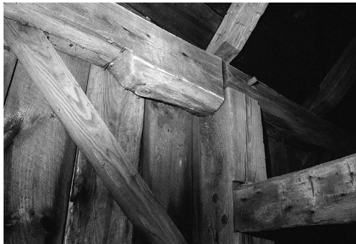
Jowled plate (one of six!) in a much-expanded 18th-century English-style barn, Huntington, Massachusetts.
