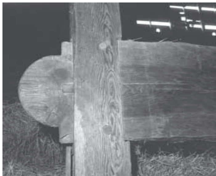
This unusual tenon profile appears on three Dutch barns in Coeymans, N.Y., likely the signature of a particular builder.
