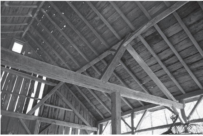
Mid-19th-century Hinsdale, Massachusetts, barn before dismantling. The continuous purlin plate assembly is canted perpendicular to the roof, and the purlin plate is flush with the roof. The rafters tenon into both upper and lower faces of the purlin plate.
