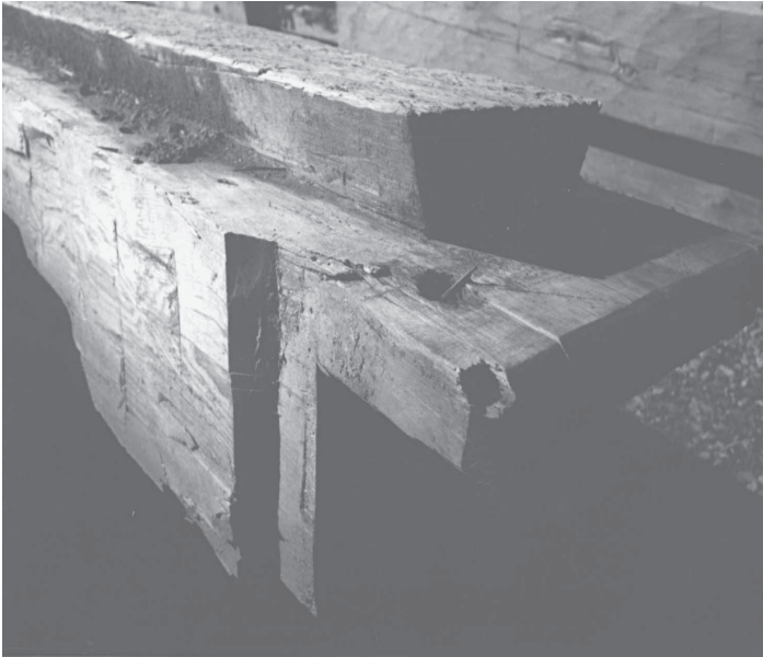
Sixty-ft. 14x17 hemlock sill girder from a barn in Middleburg, N.Y., rabbeted and undercut on both sides for 3-in. threshing-floor planks. Girder was blind-tenoned to gable sill and secured by three pins.
