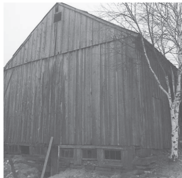
Boarding lapped at tie beam.
