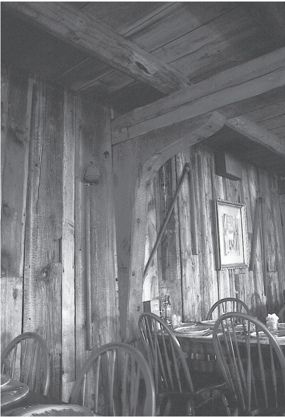
To conserve headroom, knees were used in buildings as well as ships. Cut from naturally curved, tough root-trunk or trunk-branch portions of the tree, they were pinned or bolted to the post and crossbeam. This one stiffens a Kennebunkport, Maine, gristmill and restaurant.
