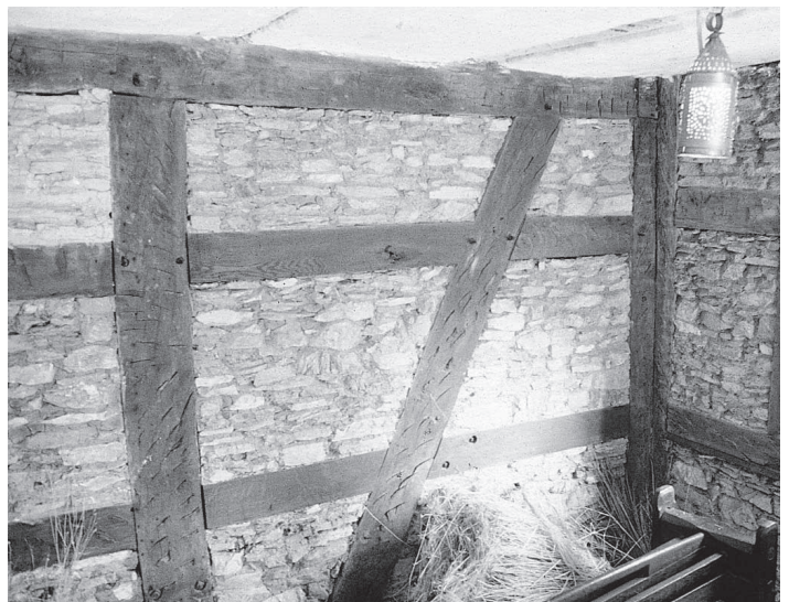
In Dutch houses with closely spaced wall posts, builders might use passing braces to achieve a long (and so more effective) brace length. In this house undergoing renovations in Alford, Massachusetts, the brace passes one post where it is lapped its full thickness and secured with a pin. Below, in lieu of normal braces, some German carpenters would angle a stud to serve as both brace and stud, as in this structure in Ephrata, Pa.
