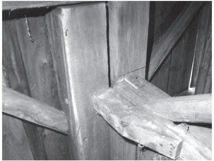
When the builder added to this barn in Savoy, Mass., he saved on a new 30-ft. tie beam by framing a piece into the post and pinning and nailing it to the existing barn's tie beam. Sheathing remains in place below tie beam; shallow wedge for dovetail tenon emerges on surface.
