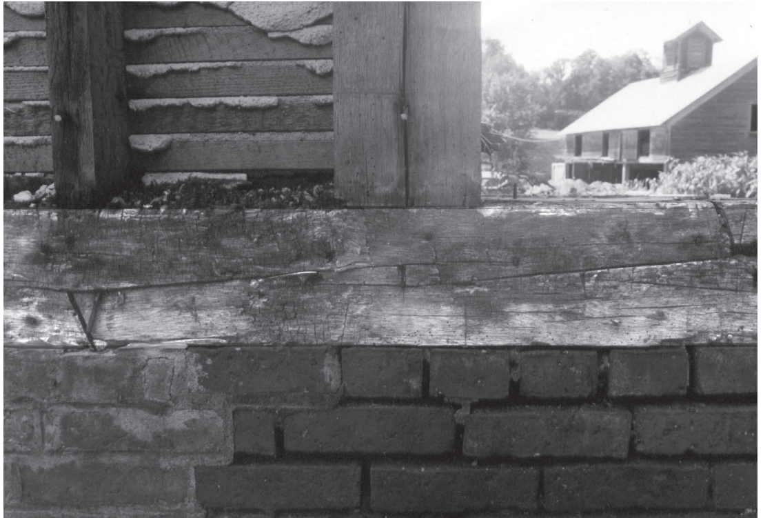
At top, bladed scarf with key, barn sill in Woodford, Calif. The sill is 8x8 Ponderosa pine, the scarf only 16 in. long. Top right, a bladed scarf used to repair a 7½ x 9½ post in a barn in Buskirk, N.Y. The tenons are 1 in. thick and 1 in. long, the scarf 23 in. long, with four pins. Above, a stop-splayed, undersquinted and tabled scarf with key used in a 6½ x 13 truss chord in the 1796 Cabildo in New Orleans (roof burned 1988, reconstructed 1992). There is barely a splay, and two forged iron straps still hold the joint together. At right, this unusual stop-splayed, undersquinted and tabled scarf in Pine Plains, New York, did not employ a key: the halves had to be slid together sideways.
