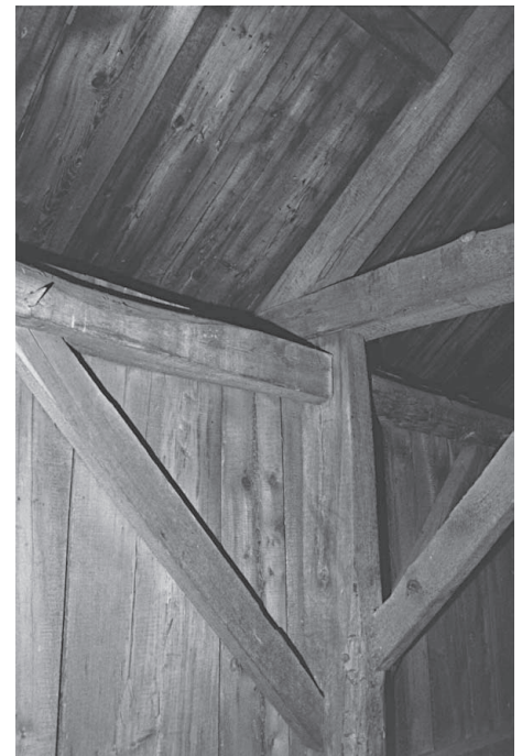
English tying joint tradition lives on after a fashion, with dropped, interrupted plates, in this Newfields, Maine, aisled barn. The plates tenon into the sides of the post; a flying plate (not visible) is supported by the tie beam ends.
