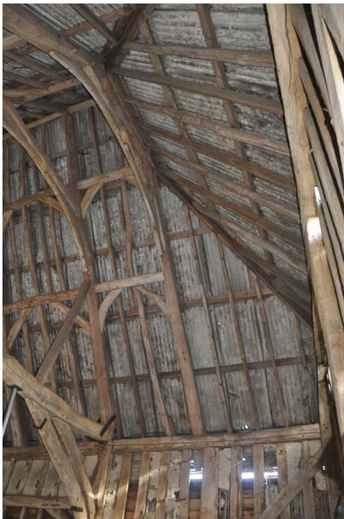
Bay 1- Roof Structure
