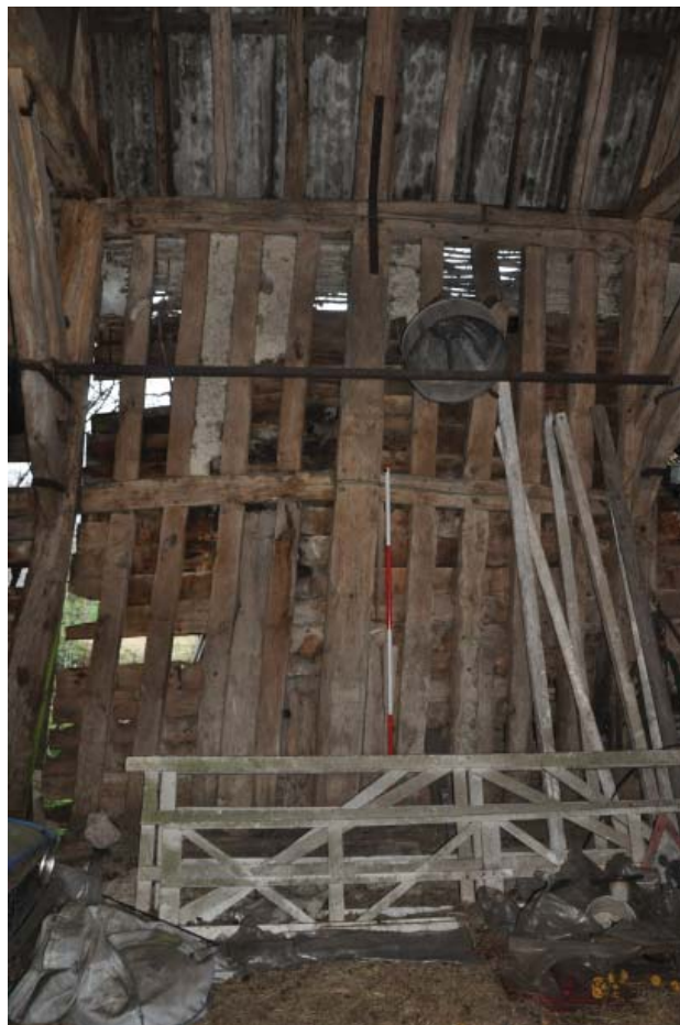
Bay 4 - A Typical Section of Wall Frame
