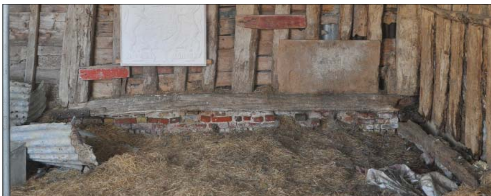
Most Intact Section of Footing and Sill Beam
