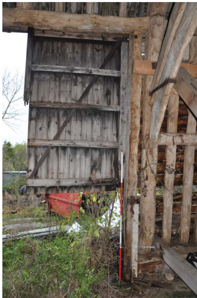
Doorway 1 Northern Post and Door
