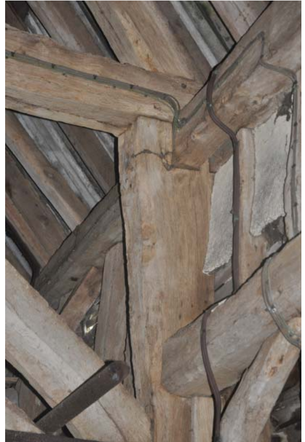
Truss 2 Eastern Post, Tie Beam and Rafter Joint
