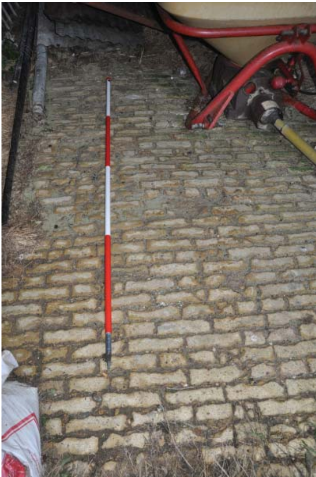
Sample of Flooring
