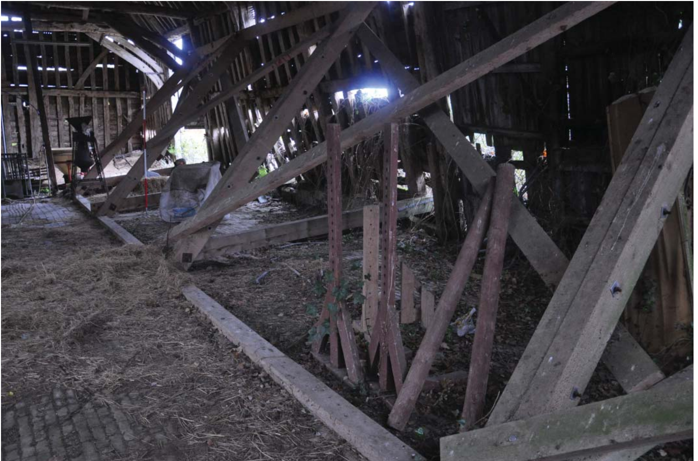
Prop work holding up the West Side of the Barn
