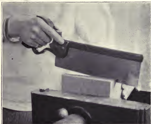
Fig. 193. Sawing the box apart.
