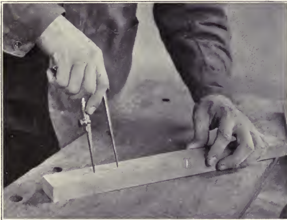
Fig. 58. Stepping off distances with the dividers
