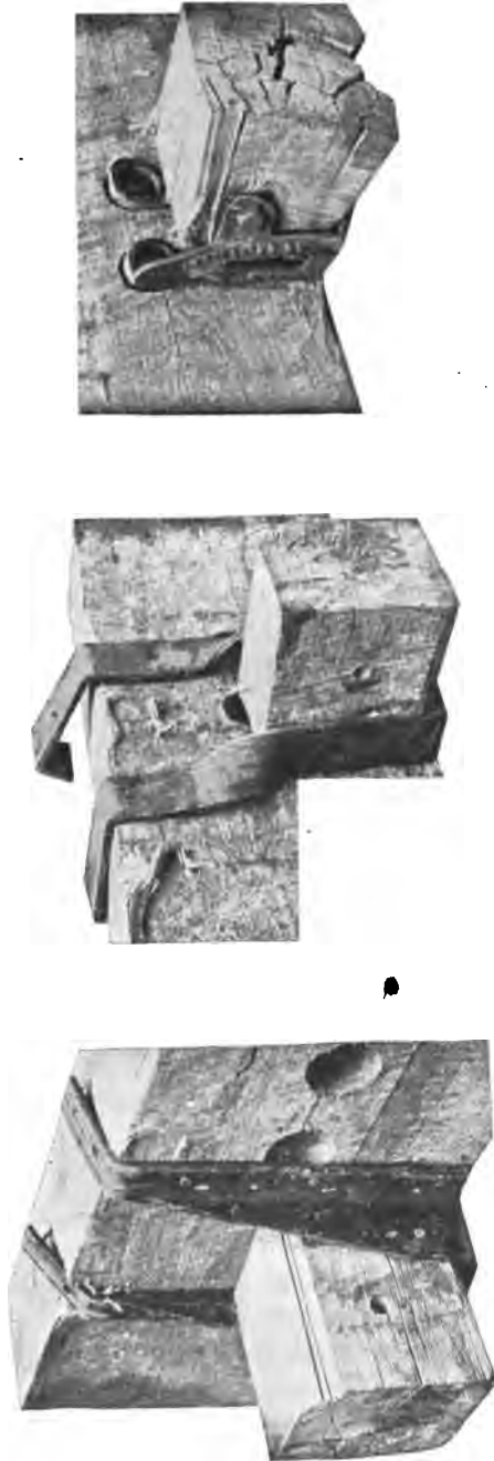
FIG. 87. JOIST-HANGERS AFTER TESTING.
